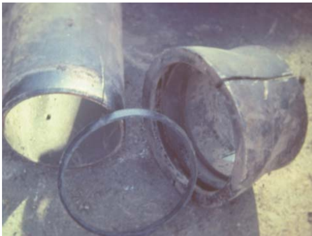
Improper Bedding Caused This Cracked Bell Joint
