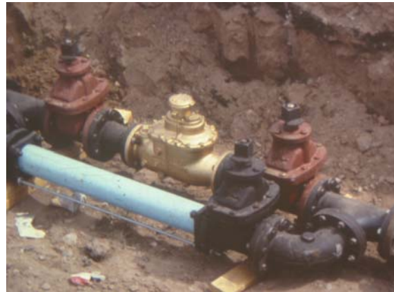
FIRE LINE INSTALLATION
